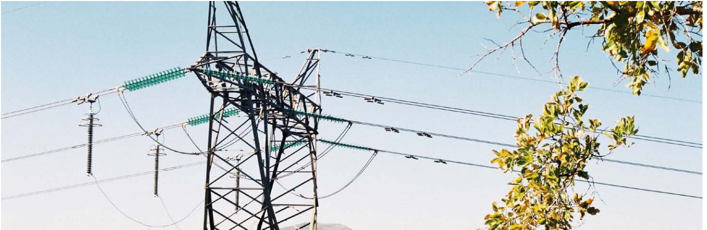
Transmission line arresters, including line discharge class 3 PEXLIM Q arresters and disconnecting devices on earth leads, erected on ESKOM 300 kV system in South Africa.
